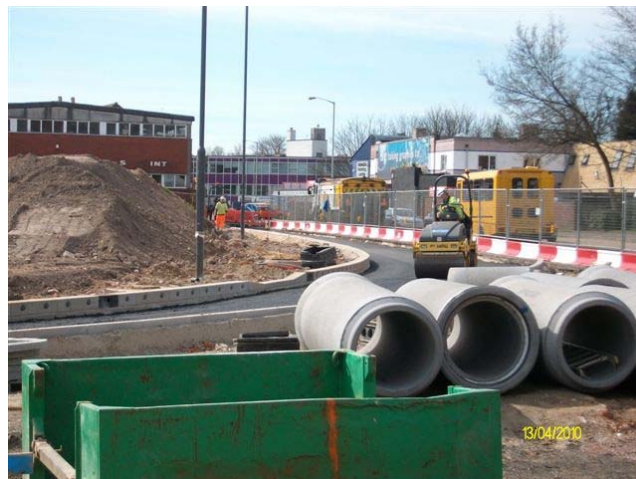
Looking south at new junction of link road with Pitt Street
